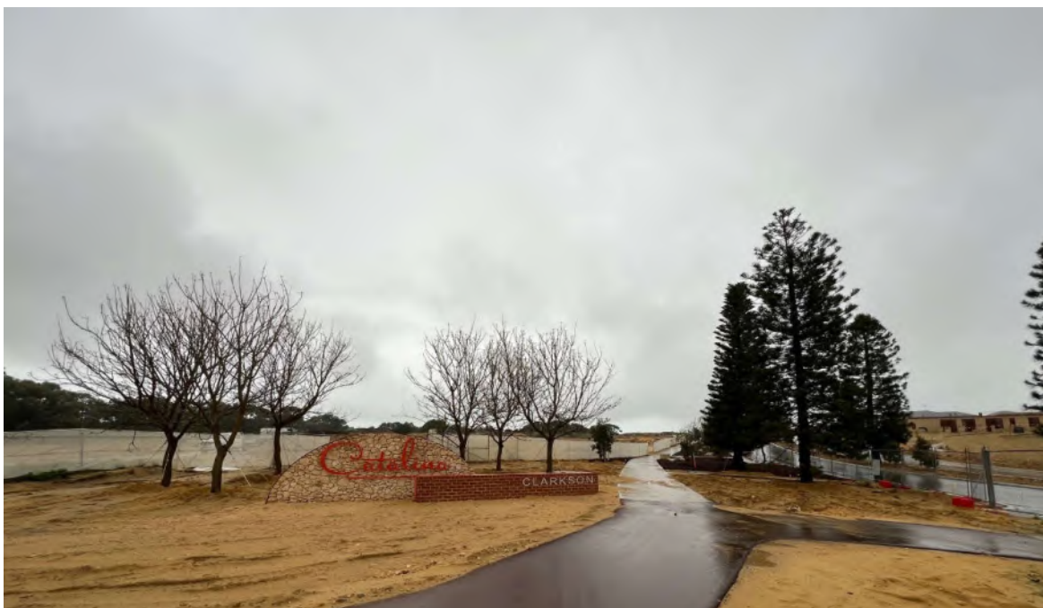
Connolly Drive/Aviator Boulevard Entry Statement construction work in progress – Catalina Central
