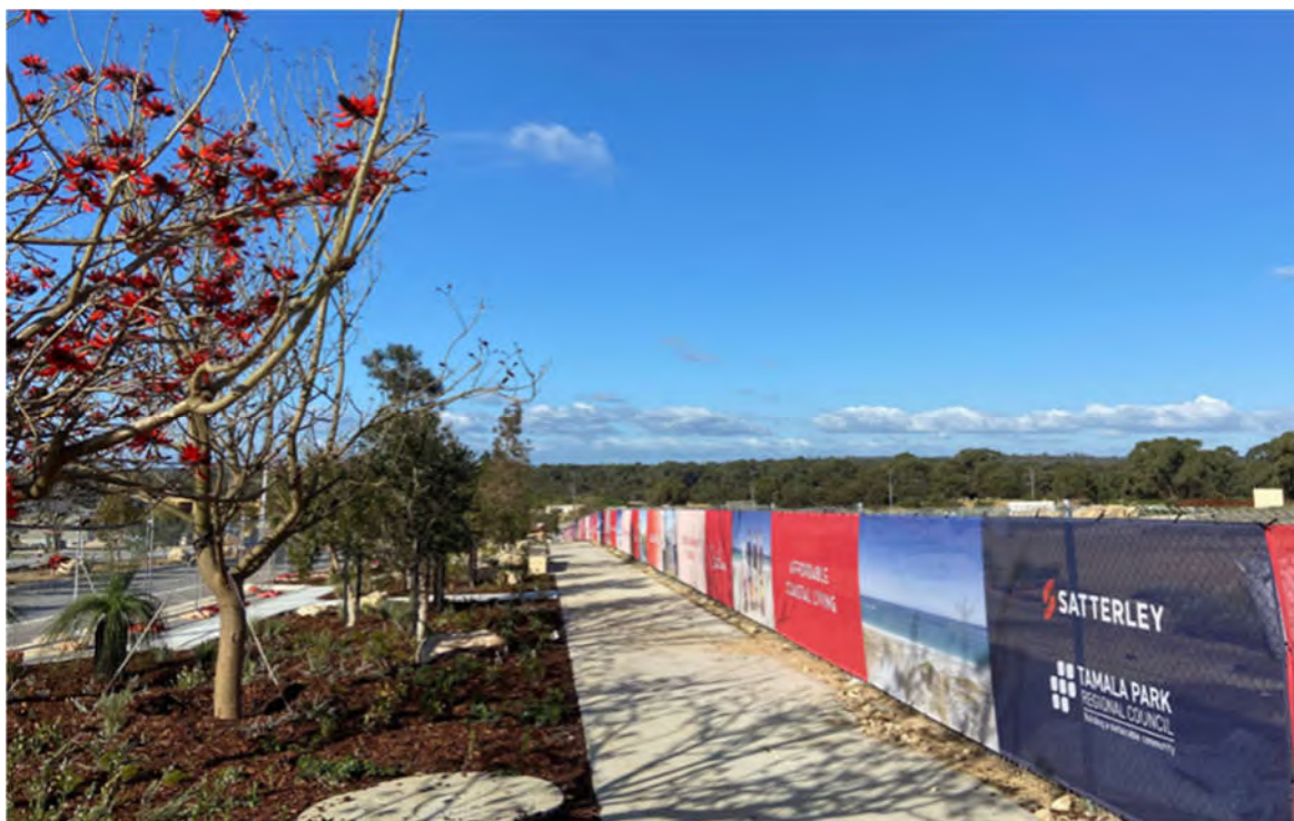
Greenlink landscape construction work in progress – Catalina Central
