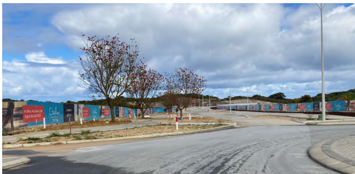
Portofino Promenade Landscaping – work in progress
