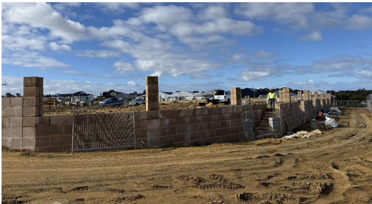
Stage 44 civil works in progress
