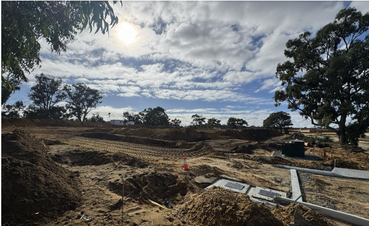
Stage 47 civil works in progress
