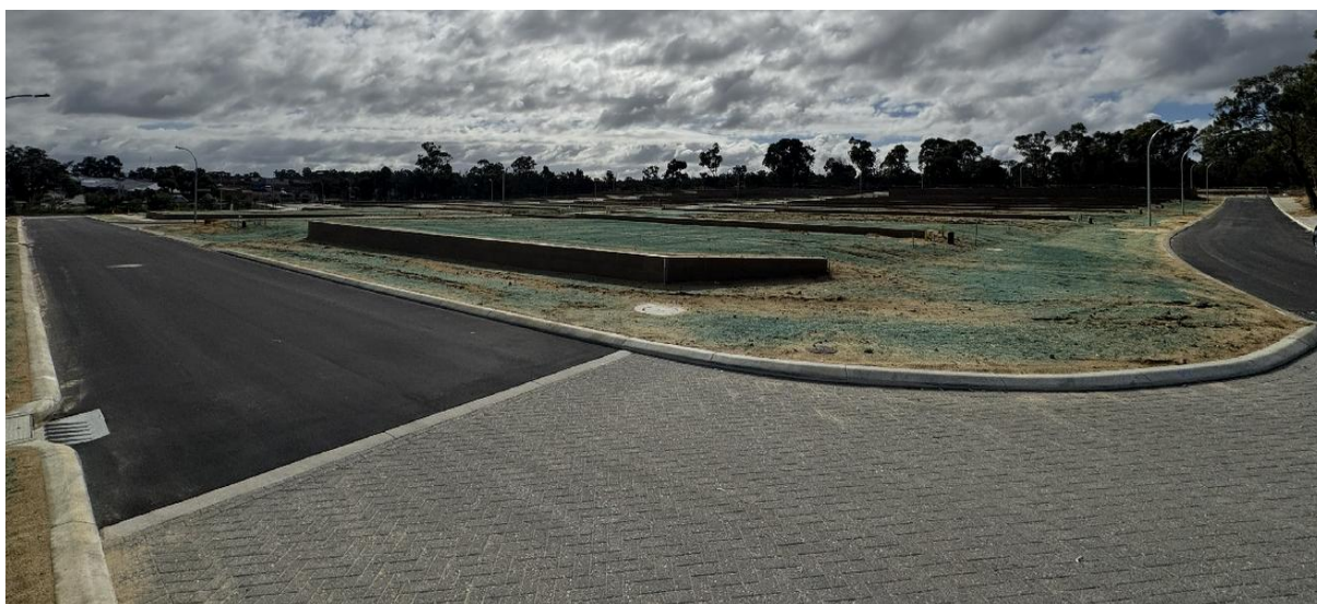
Completed Stage 45 civil works
