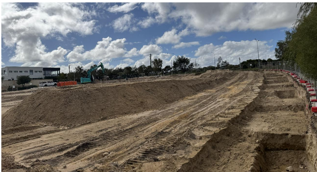
Stage 51 civil works in progress
