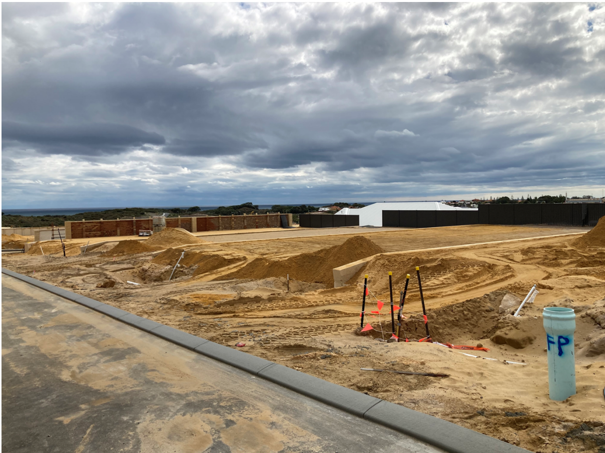
Stage 29 civil works in progress
