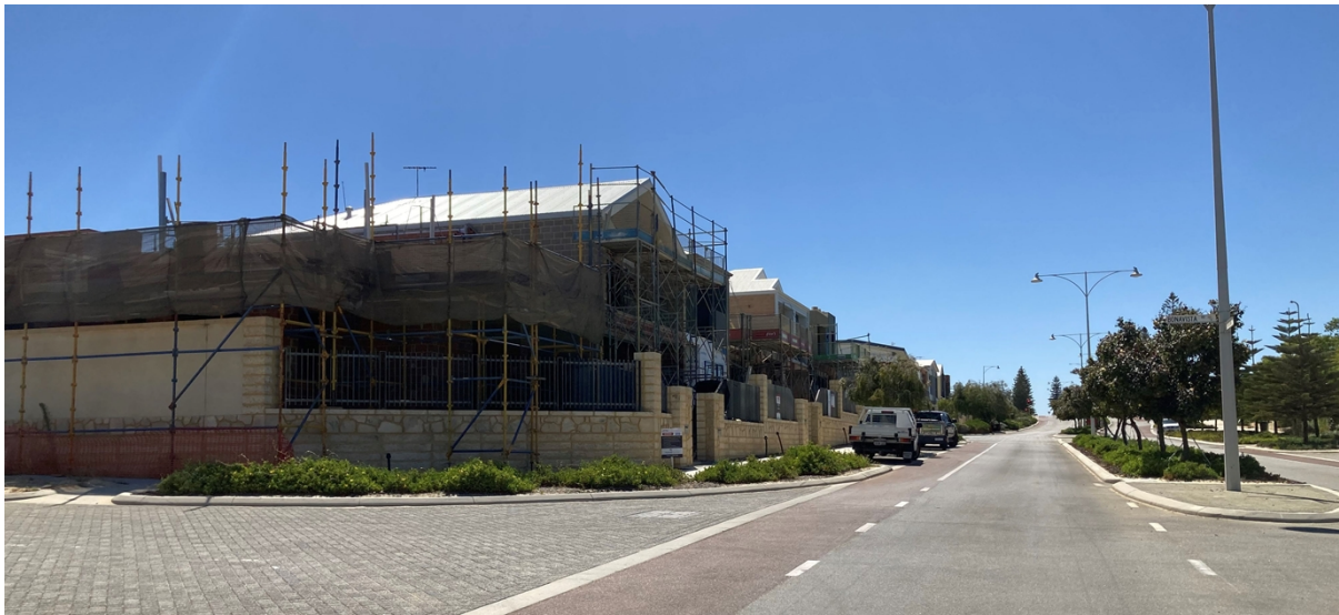
Double-storey homes under construction on Portofino Promenade in Stage 27 - Catalina Beach
