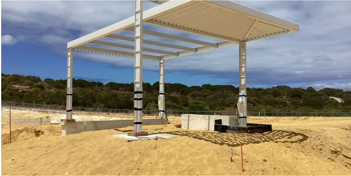
Foreshore Park under construction
