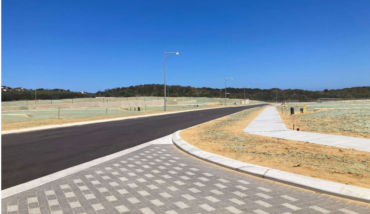
Stage 31 – Construction complete and Titles issued.
