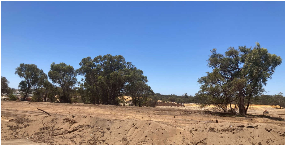
Stage 41-43 Bulk Earthworks in progress
