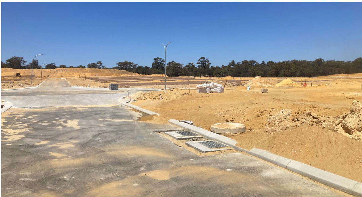
Stage 38 Civil Works in progress
