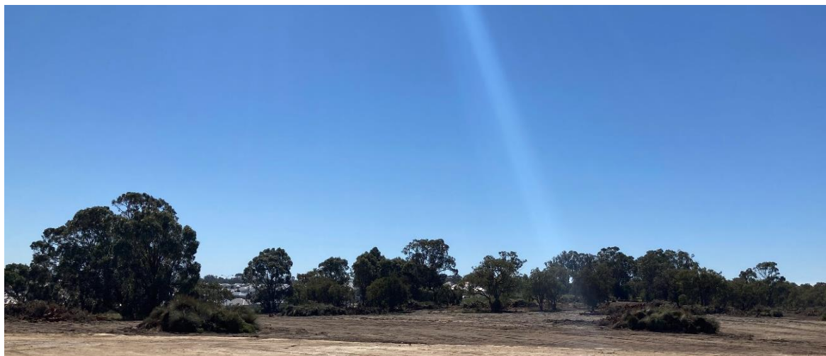
Catalina Green Earthworks in progress
