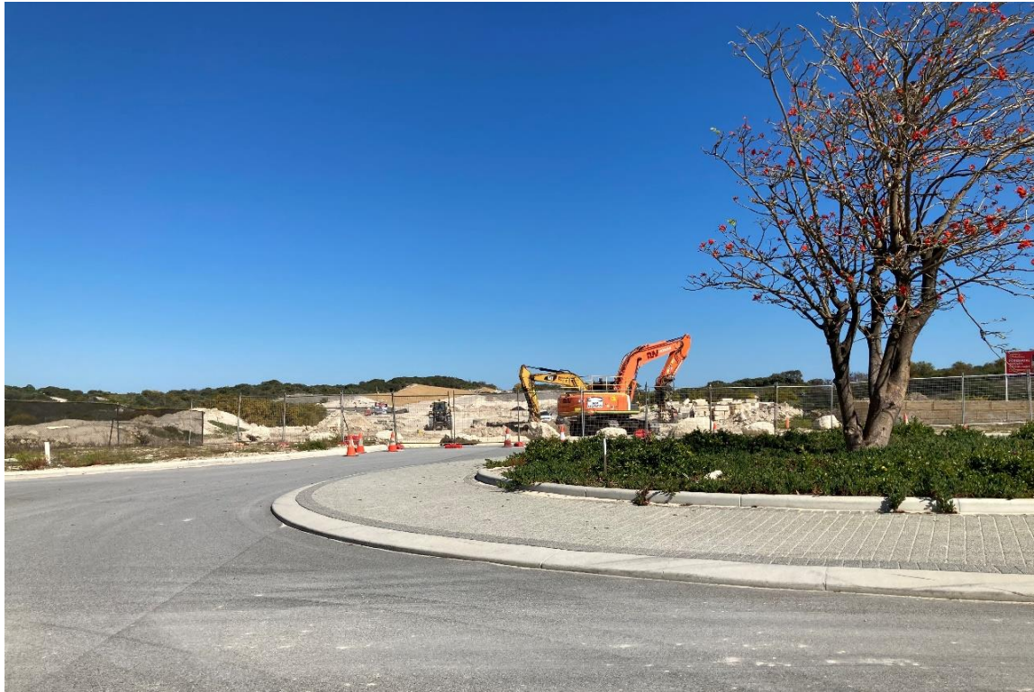
Portofino Promenade extension under construction, Catalina Beach
