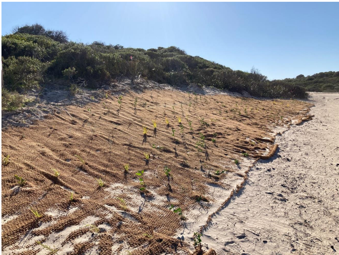
Revegetation works adjacent to the Foreshore Access Road alignment
