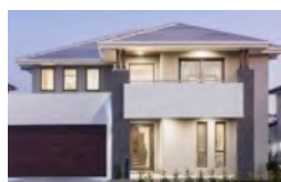
Double storey house
