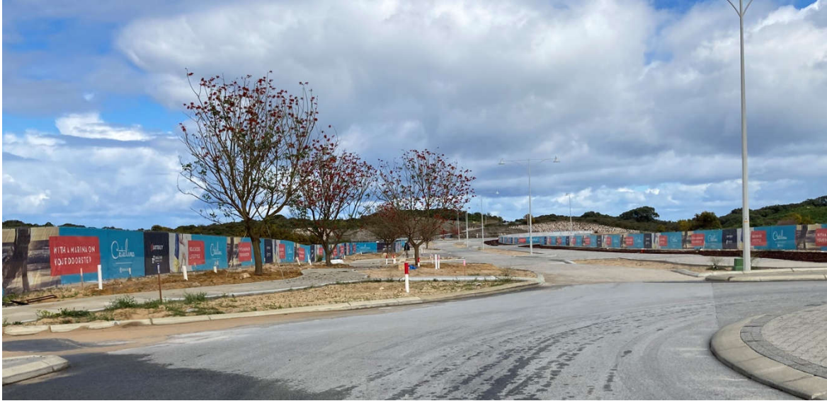
Portofino Promenade Landscaping – work in progress
