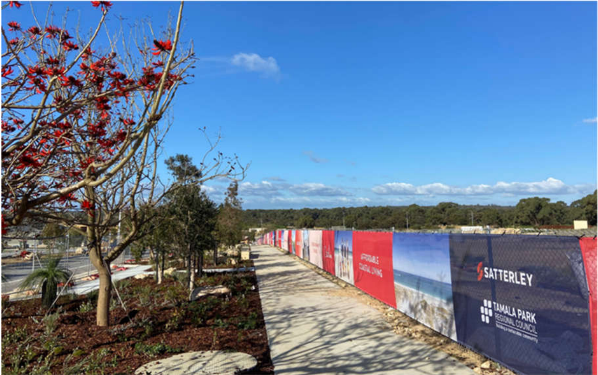
Greenlink landscape construction – Catalina Central
