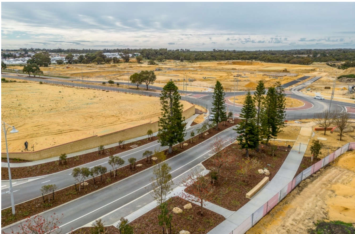
Stage 36 Civil Works and Connolly Drive Landscaping – works in progress
