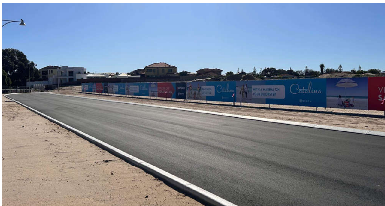
Completed Longbeach Promenade extension – looking north
