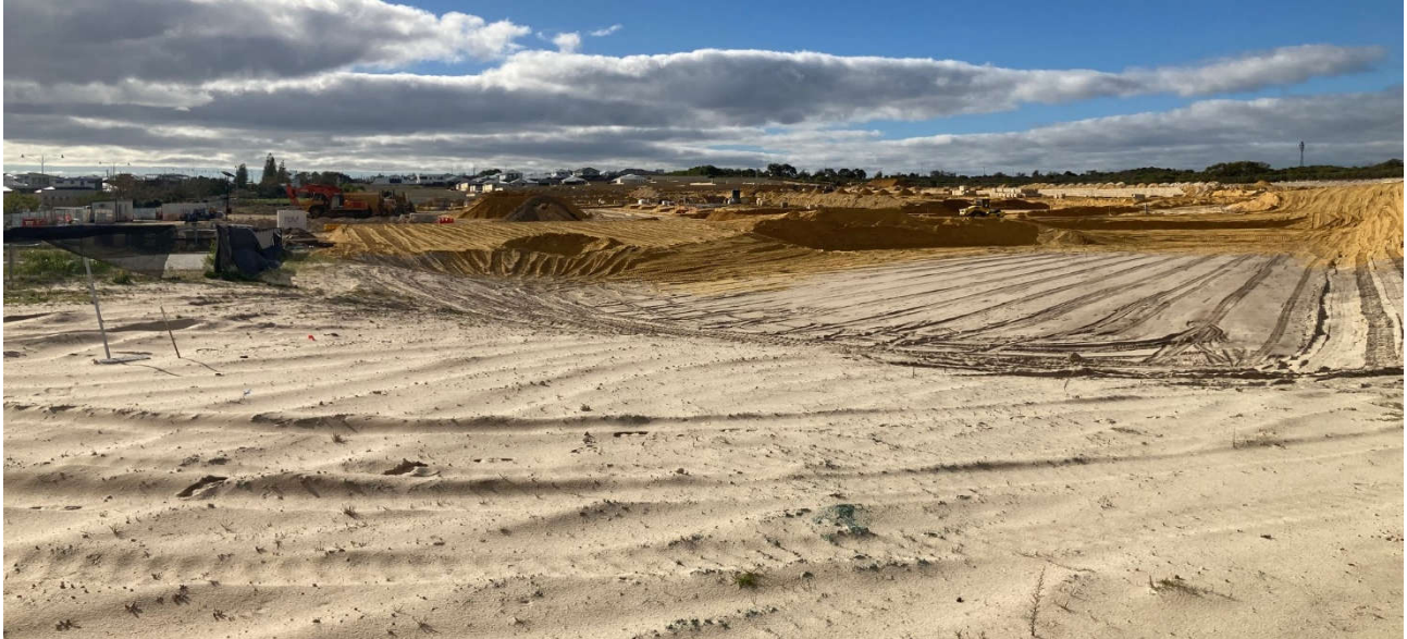
Stage 31 Earthworks (looking east) include Foreshore Park and drainage basin preparation
