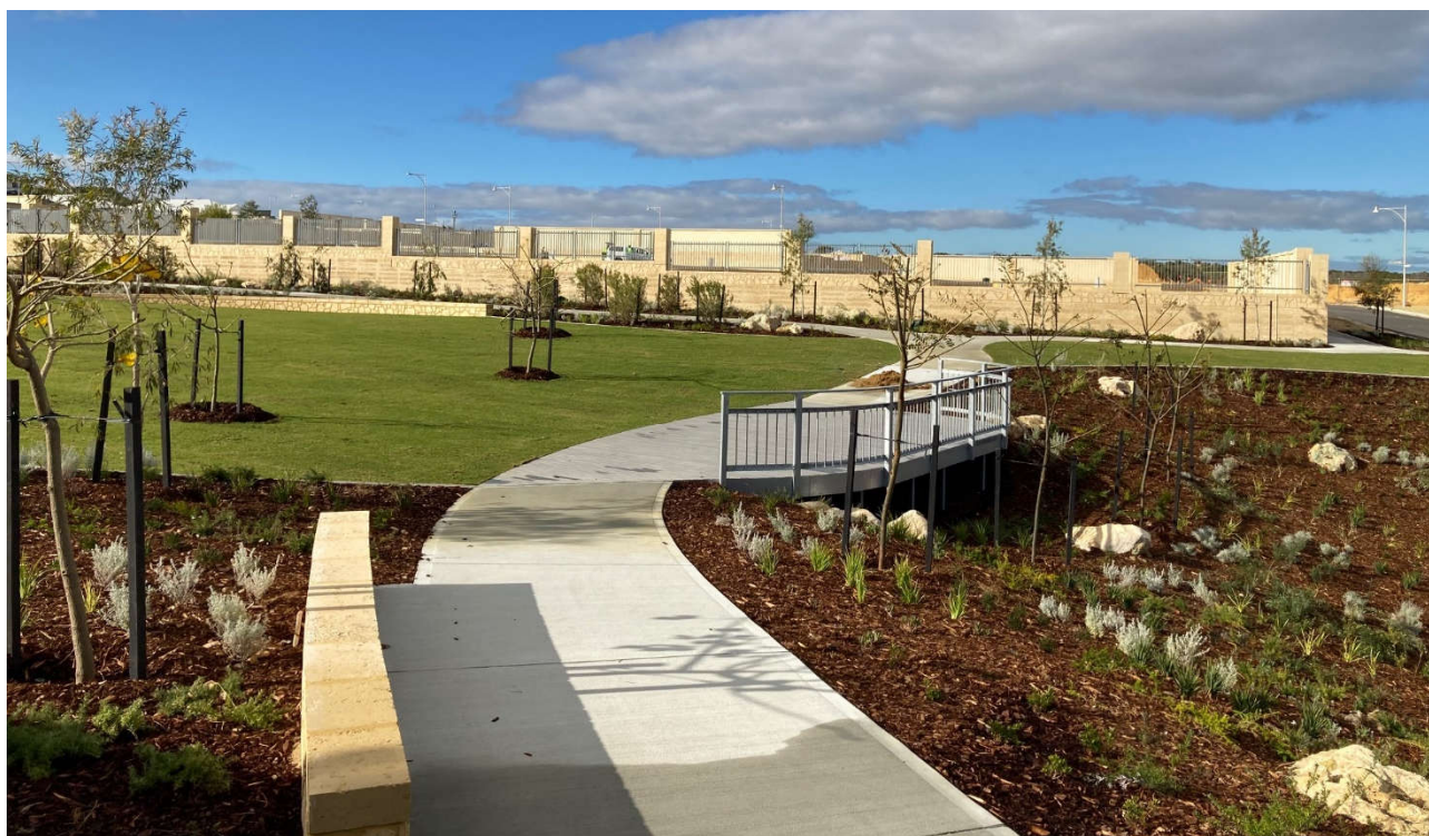
Stage 25 Phase 2 Park works – nearing completion
