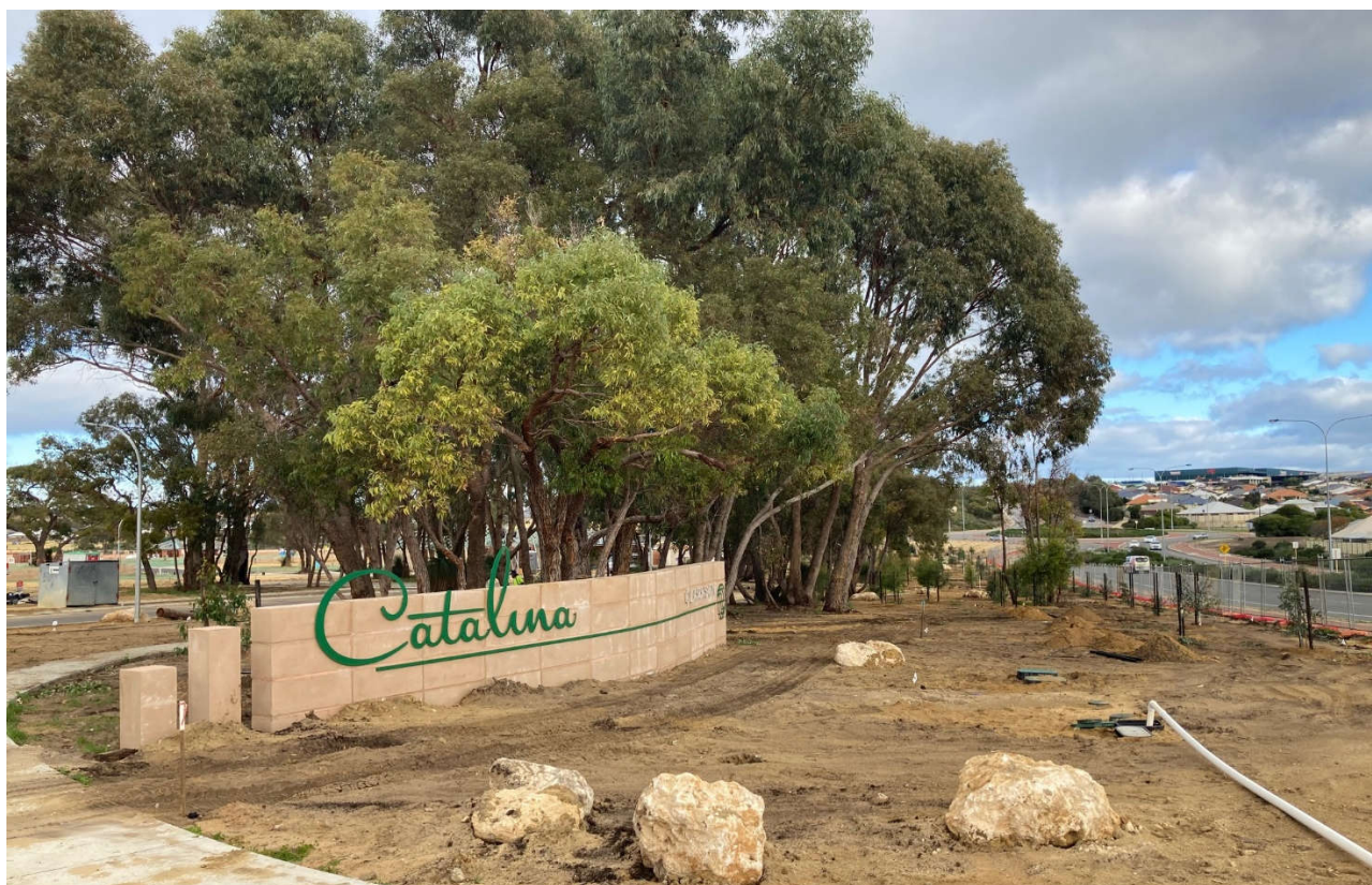
Stage 36 Park works in progress – adjacent to Neerabup Road, looking west
