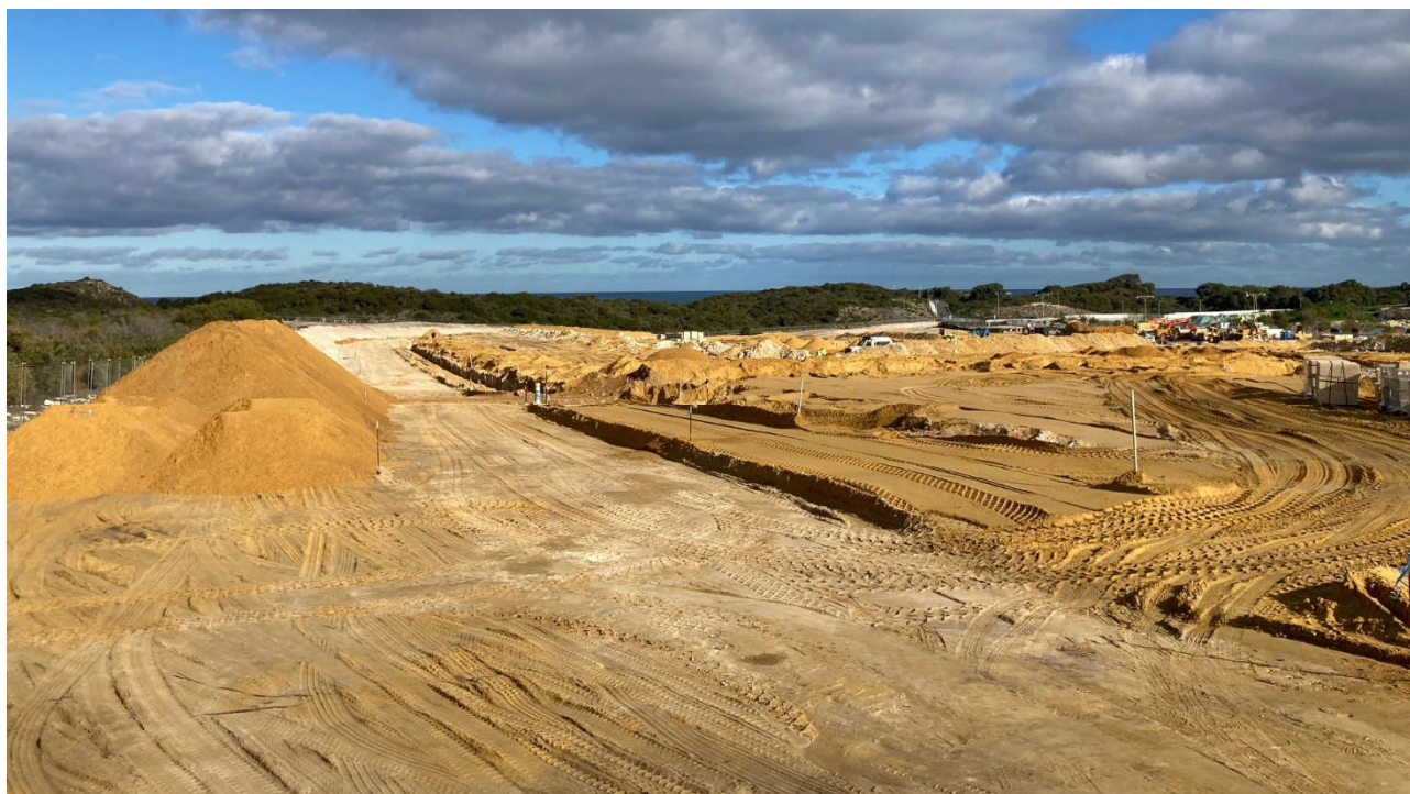
Stage 31 Civil Works in progress
