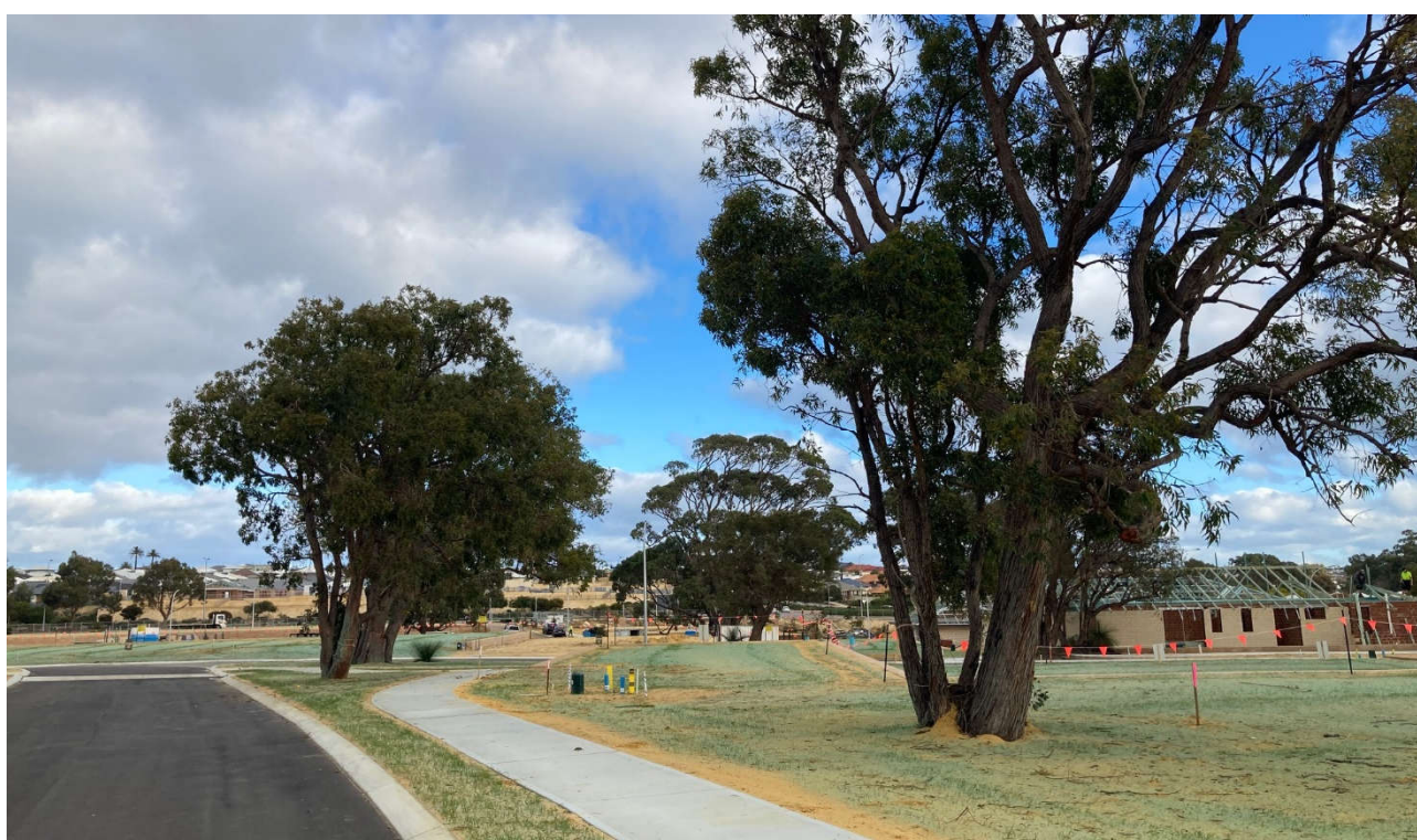
Completed Stage 37 Civil Works
